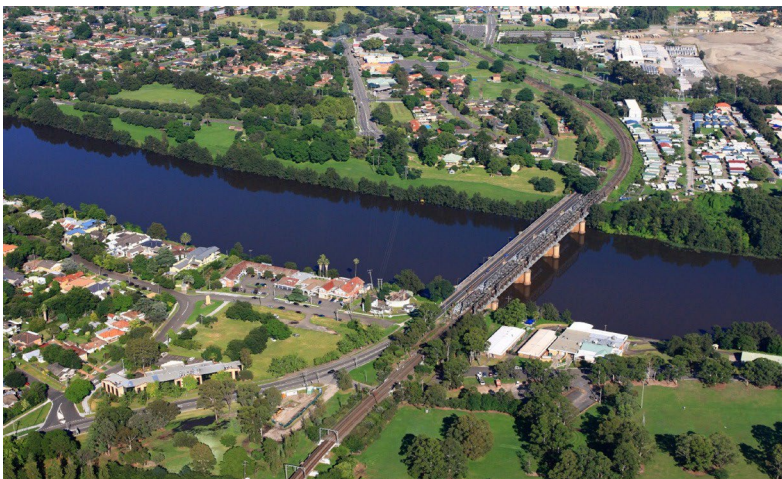
Aerial photo of the Emu Plains Primary Mains Extension.
